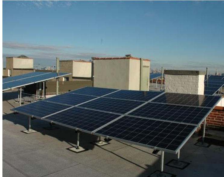
MECHANICALLY ATTACHED PLANAR ARRAY
