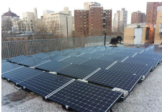
Low-profile ballasted mounting system
