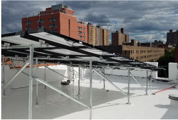
Mechanically attached mounting system
