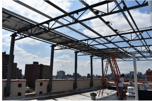
Elevated solar canopy, mid-installation
